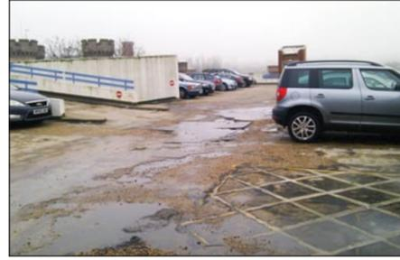
The multi-storey staff car park at Leicester Royal Infirmary had fallen into a critically bad state. Years of exposure to the elements and to de-icing salts had caused widespread delamination on the top deck, leaving large sections of the steel reinforcement completely exposed.
