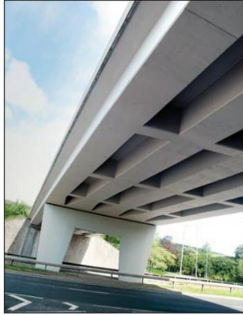
West Dunbartonshire Council has specified a concrete repair system from **Sika** to refurbish the Mountblow flyover in Clydebank, which was suffering from corrosion due to years of carbonation and chloride attack.
