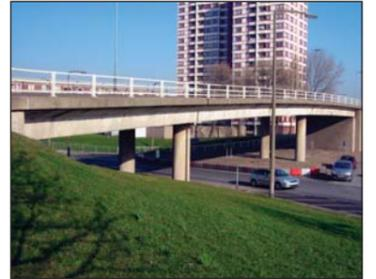
When the steel reinforcement of the concrete Balby Flyover began to suffer from corrosion, due to carbonation and chloride attack, Doncaster Council required a reliable renovation method that would not only provide long term protection, but would also enable the bridge to remain open during repair operation.
