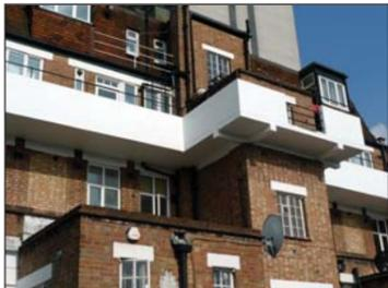
Constructed in the 1930s, the rear walkway balconies to Croydon's Victoria House had become extremely dilapidated and in urgent need of remedial repairs.
