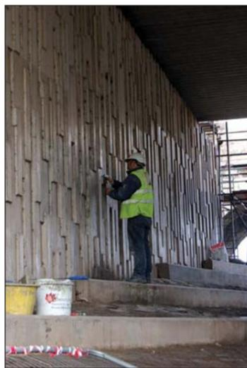
Extensive concrete repairs, as well as the design and installation of electro-chemical works (permanent monitoring and cathodic protection trials) have been carried out at **Cliff Gardens Bridge**, in Old Colwyn, by CRA member **Quadriga Concepts Ltd**.
