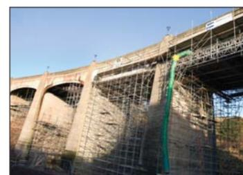
CRA member, **Freyssinet Limited**, is currently working on a £1.5m contract for repairs to the **A92 Jubilee Bervie Bridge** near Montrose, Scotland. This 1930s reinforced concrete structure has suffered the ravages of the marine environment and extensive repairs were required.
