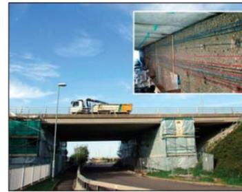
Principal Inspection reports on the two bridges at **Tipner Interchange** in Portsmouth revealed leaking joints above the two intermediate piers on each structure. Subsequent testing work confirmed the presence of very high chloride concentrations in the piers.
