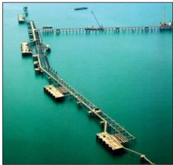
The South Hook LNG development in South Wales; the biggest natural gas terminal in Europe, has undergone a massive refurbishment and refit. A key element was substantial repairs to the 40-year old jetty, including strengthening of existing piles and large amounts of concrete reinstatement.
