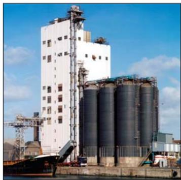
Due particularly to the chloride containing marine atmosphere, the 75 metre high, 13,500 tonne capacity, monolithic concrete grain silo at **Lowestoft Docks** had been suffering from cracking and spalling, with the consequent water ingress accelerating the deterioration.
