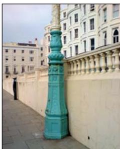
Over the years some of the top spigot sections had worked loose within the bottom socket section of each post and required 'tightening up'. This was achieved by drilling through the cast iron base into the gap and injecting with Sika Rail KC330, a 2-part flexible resin normally associated with stabilising track in the rail industry.
