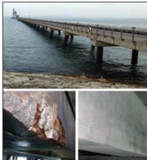
The offloading jetty is an essential asset for Anglesey Aluminium as it enables them to take delivery of raw materials directly into its UK aluminium processing facility. Being exposed to the harsh environment of the sea, the natural presence of salt had contaminated the concrete and caused corrosion of the steel reinforcing bars.
