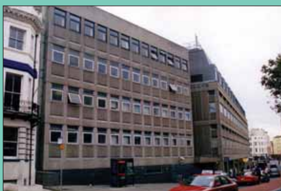
The Hastings building before repair work (and detailed investigation)
