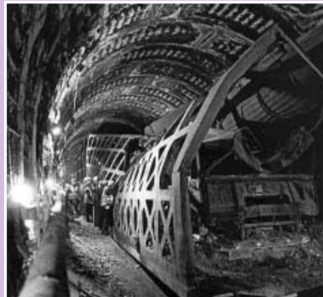
Above: Typical depth of spalling following a fire.
