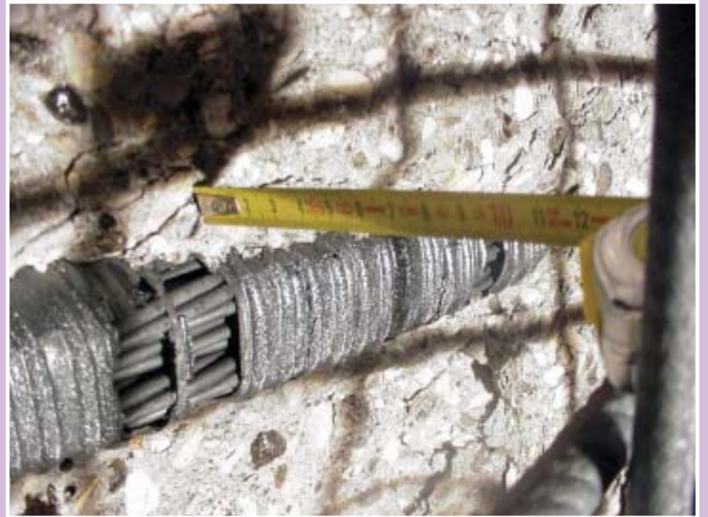
Above: Typical depth of spalling following a fire.
