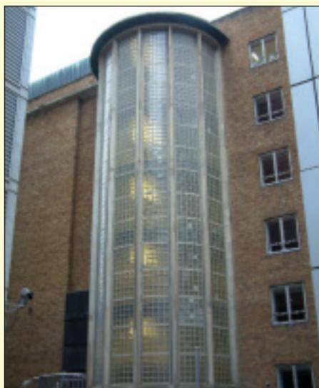
Yoldings have won the Science Museum contract for Concrete Repairs to the staircase columns. On site now, the contract also involves replacement of damaged glass bricks to the structure – no easy feat, as the bespoke nature of the bricks involved manufacturing new dies. Repairs are being effected using the WeberSBD Mulsifix system.
