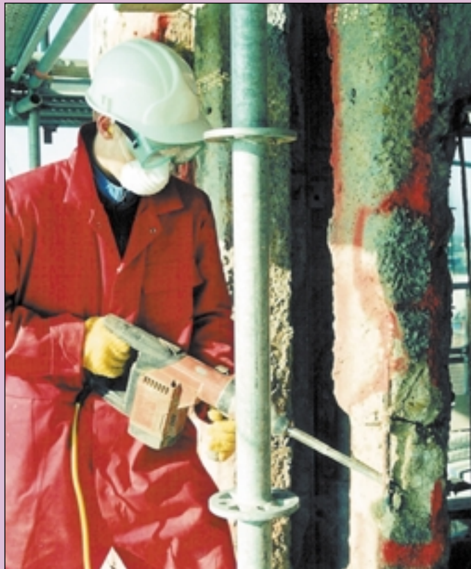
Picture by kind permission of CRA member, Concrete Repairs Ltd.
