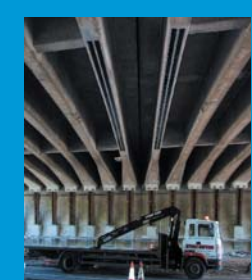
M62 J21 Ashfield Bridge
