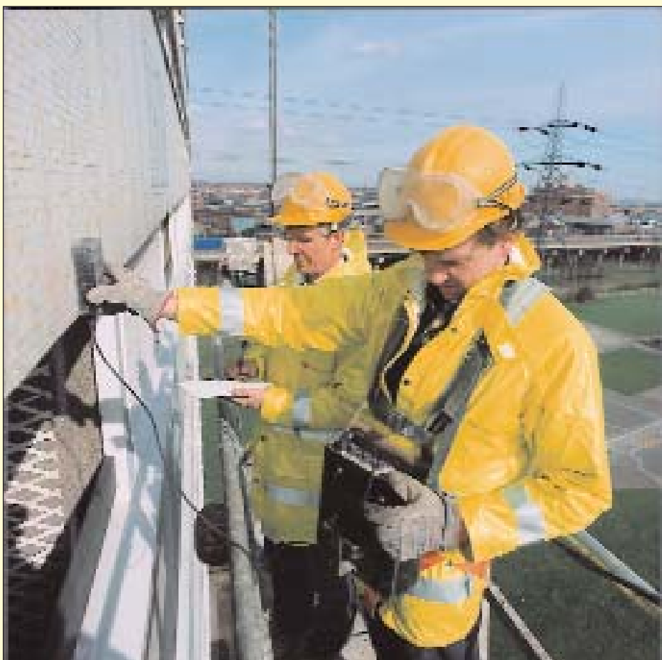
Early survey work essential says the CRA.
