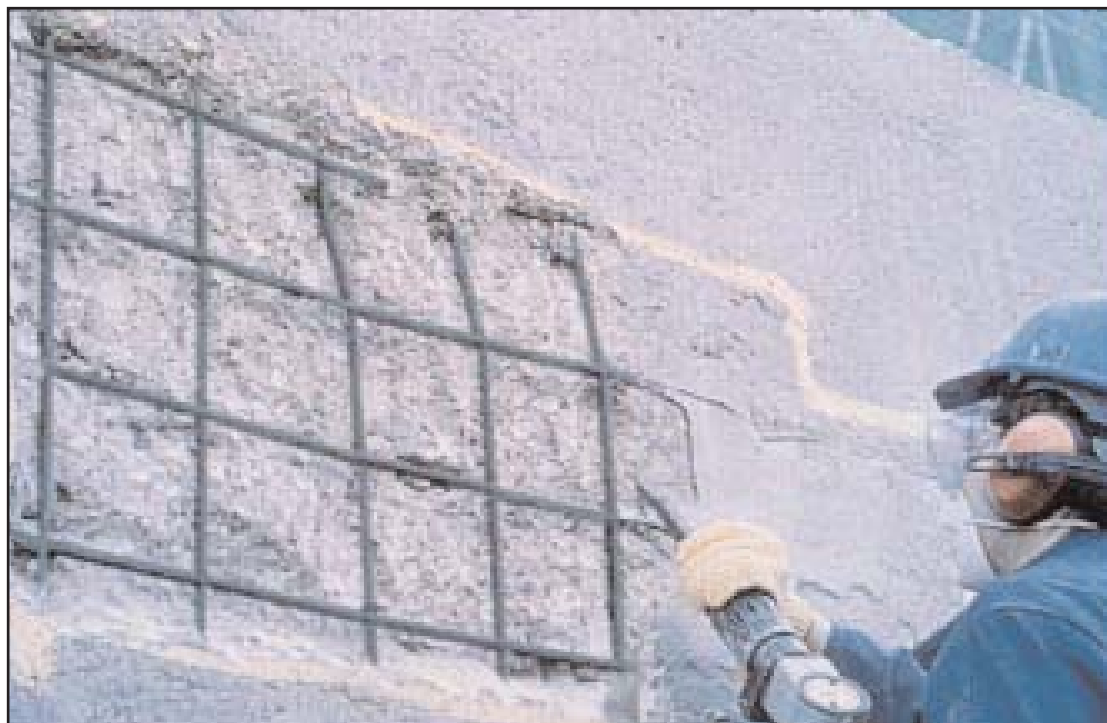
Agreed and defined areas of concrete repair are all-important.
