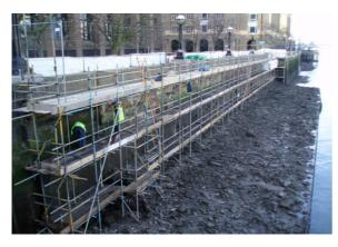
Scaffolding was progressively erected along the face of wall, founded on the riverbed and mechanically tied to the wall, with all scaffold boards tied down to prevent movement due to tidal action.
