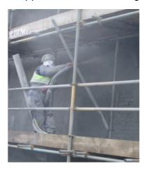
This was followed by preparation of the surfaces by grit blasting to provide a key for the application of a spray concrete containing an alkali free accelerator and reinforced with polypropylene fibres. The finish was cut to line and trowelled whilst the excess material was cleaned from the scaffold and riverbed prior to the rising tide covering the work.
