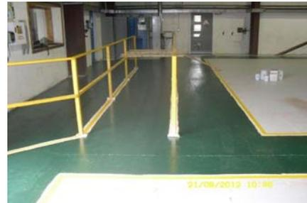
colours to allow walkways, parking bays, muster points etc to be easily distinguished from the main body of the floor. Templates can also be used to display symbols and directions such as emergency exits, first aid stations etc.
