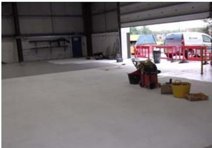
The system applied was Epoch, manufactured by Spencer Coating, Skyform are an approved applicator of all Spencer Coatings systems. The system is applied in The first stage of the flooring system was application of a stabilising primer which seals the existing surface and provides a finish for the non-slip element of the system to bond to. A non slip coating is then applied, for this project a material with non-slip aggregate premixed
