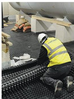
Once the swimming pool had been completed, the Cavity membrane division of Cemplas followed on to deal with water ingress in the plant rooms and vast ventilation tunnels. Using Sika's Cavity Drainage System this was applied to cover the walls and floors. Once the Cavity Drainage System had been installed, a plaster membrane was applied to the walls, and a screed incorporating a
